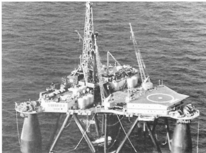
Figure 16.25 This floating oil derrick provides its own energy needs. Four diesel-driven generators rated 1200 kVA, 440 V, 900 r/min, 60 Hz supply all the electrical energy. Although ac power is generated and distributed, all the motors on board are thyristor-controlled dc motors. (Courtesy of Siemens)
